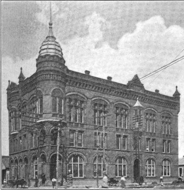
THE BANK'S BUILDING.
